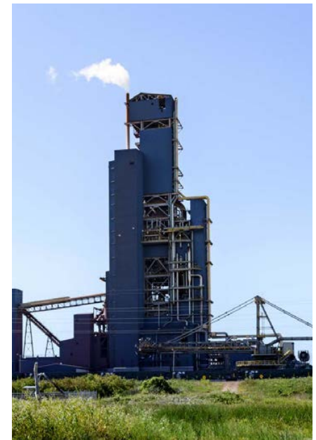
Cliff's Toledo HBI plant
