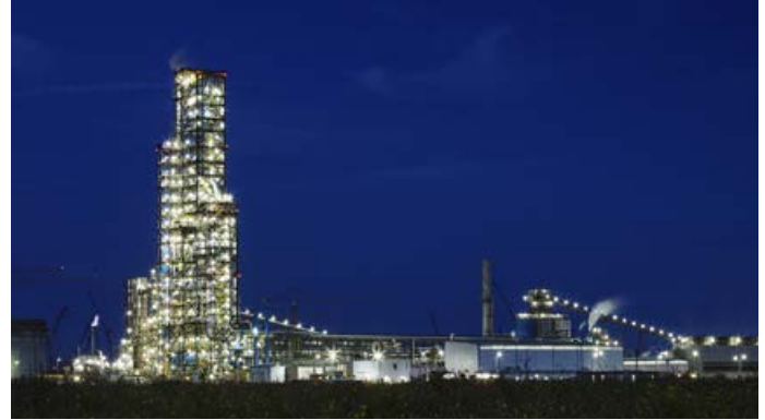
voestalpine Texas MIDREX® HBI Plant located near Corpus Christi, Texas, is the world's largest HBI plant.
