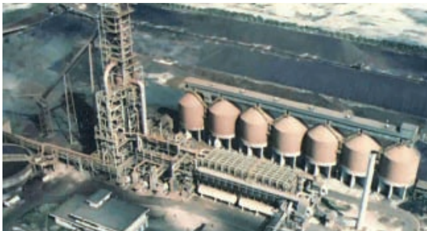
Figure 7 - Antara Steel Mills
