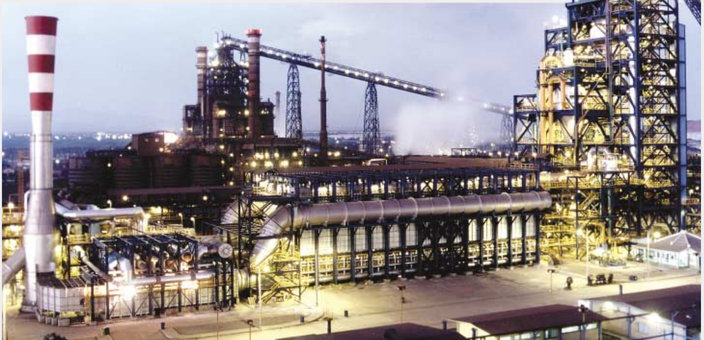
IMEXSA Plant at Lázaro Cárdenas, Mexico
